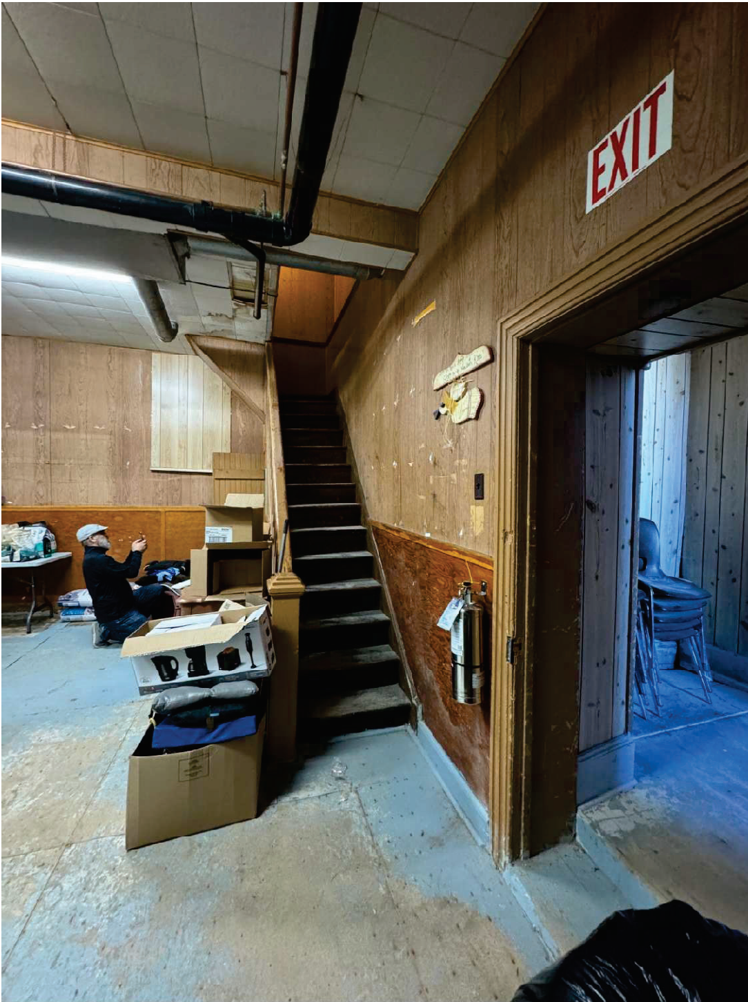
Photo #44 Basement North Exit/Access and North Stairs Leading to Ground Floor, Looking West
