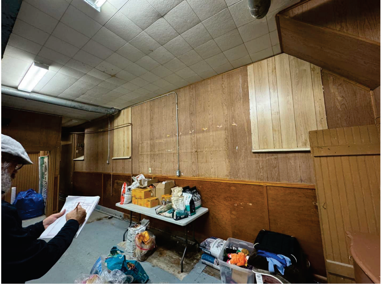
Photo #49 Basement east wall, looking west.
