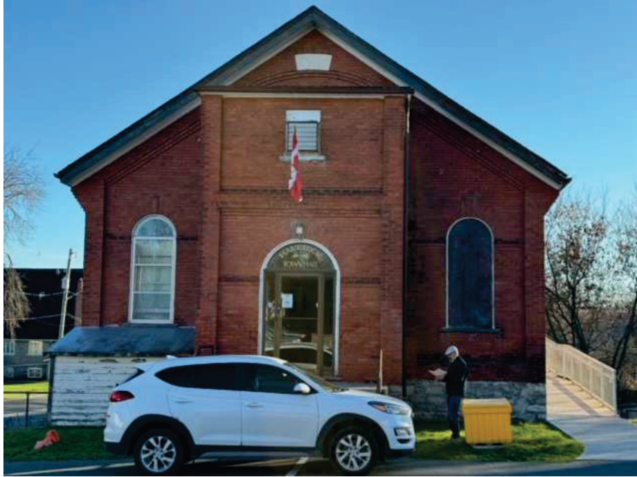
Photo #1 General View of the North Elevation
