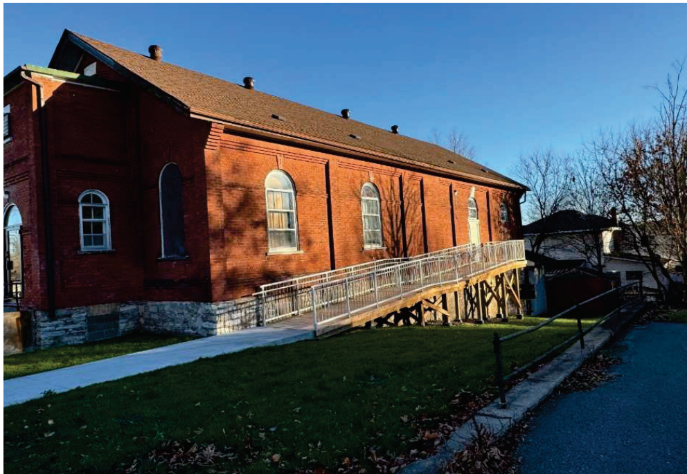
Photo #4 General View of the West-North Elevations
