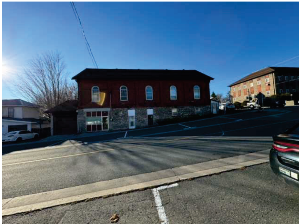
Photo #2 General View of the East Elevation
